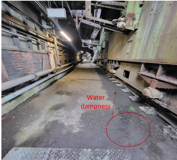
Fig 3: Water disposed around the towing vehicle IV, photo captured by Sooraj Nair, October 2024
