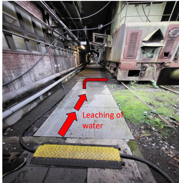
Fig 2: Water disposal way towards the towing vehicle IV and towing vehicle V. Photo captured by Sooraj Nair , October 2024
